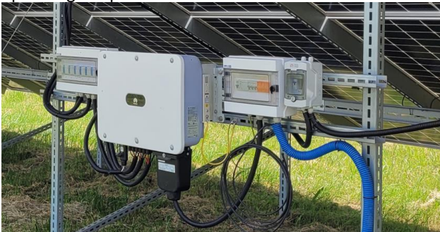
Fig. 5. Inverter and protection system in a photovoltaic installation. [own work]
